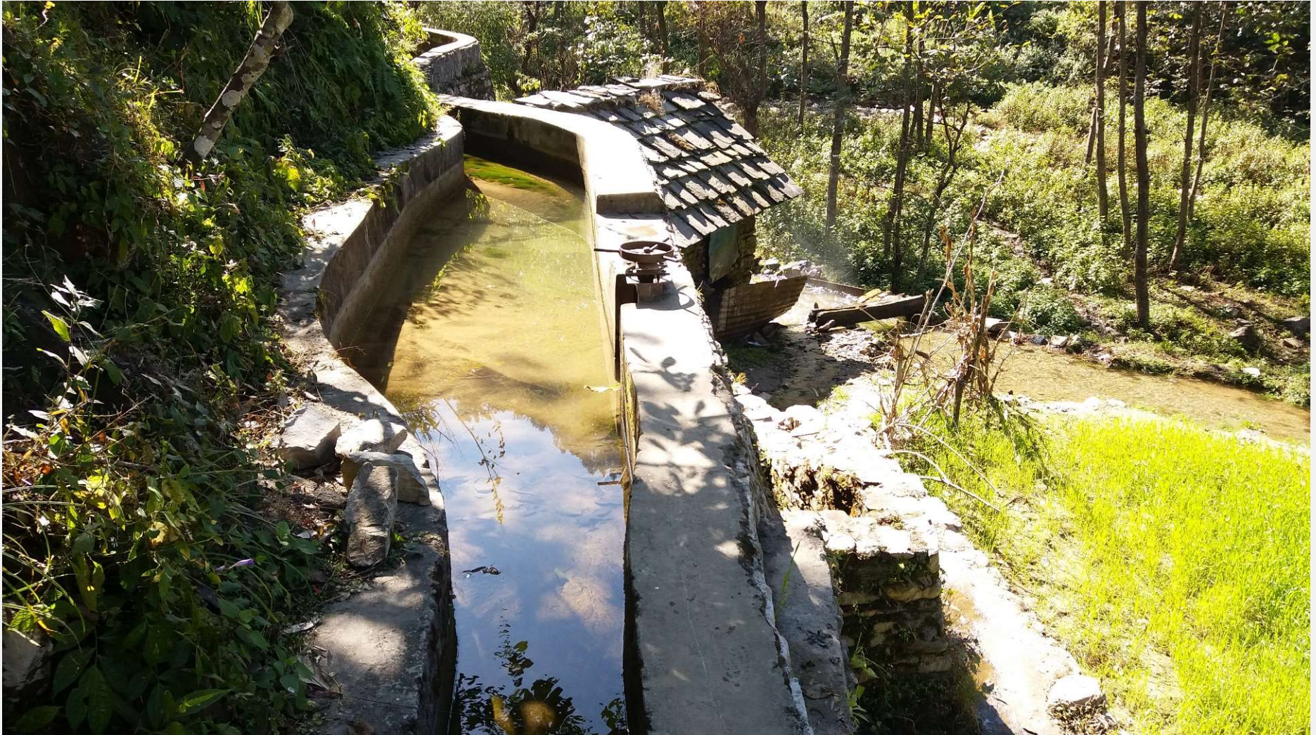
Flushing Arrangement in Settling Basin
