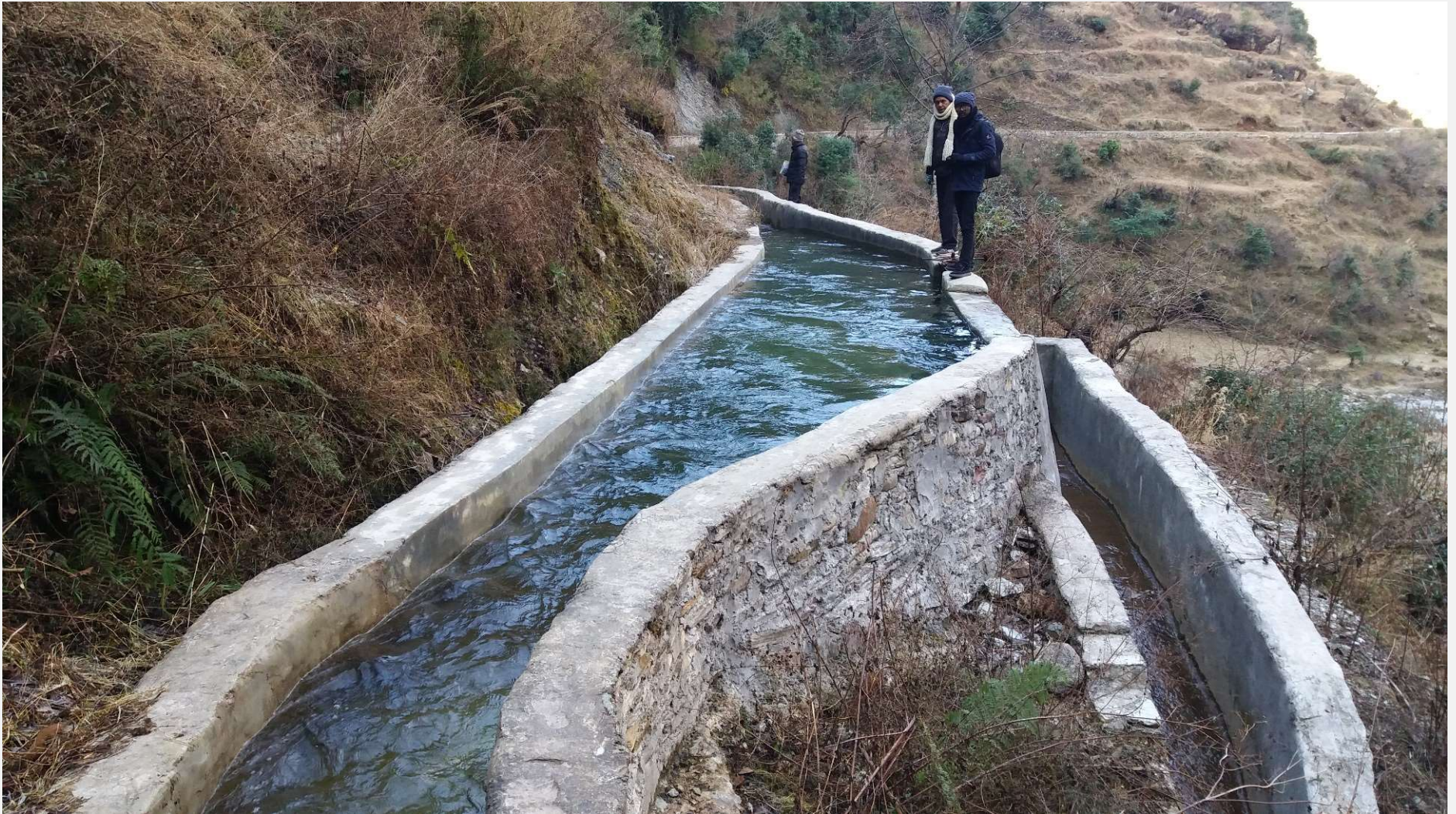
Gravel Trap/ Settling Basin
