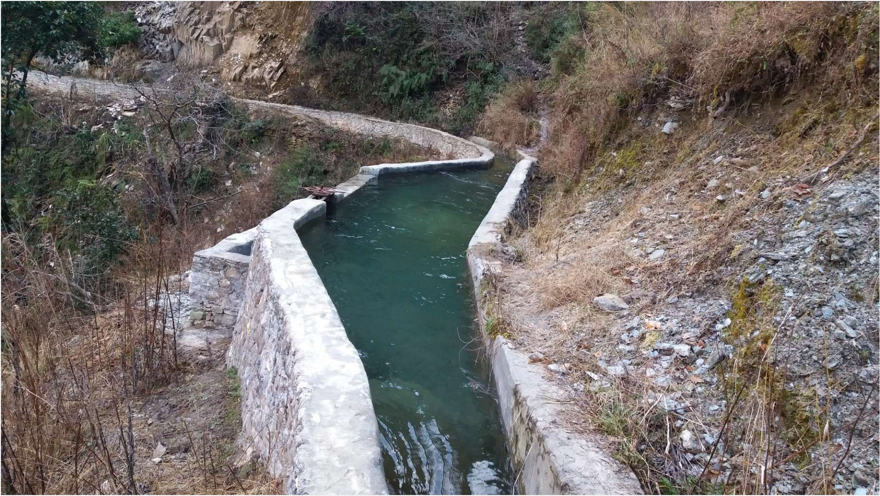
Gravel Trap/ Settling Basin
