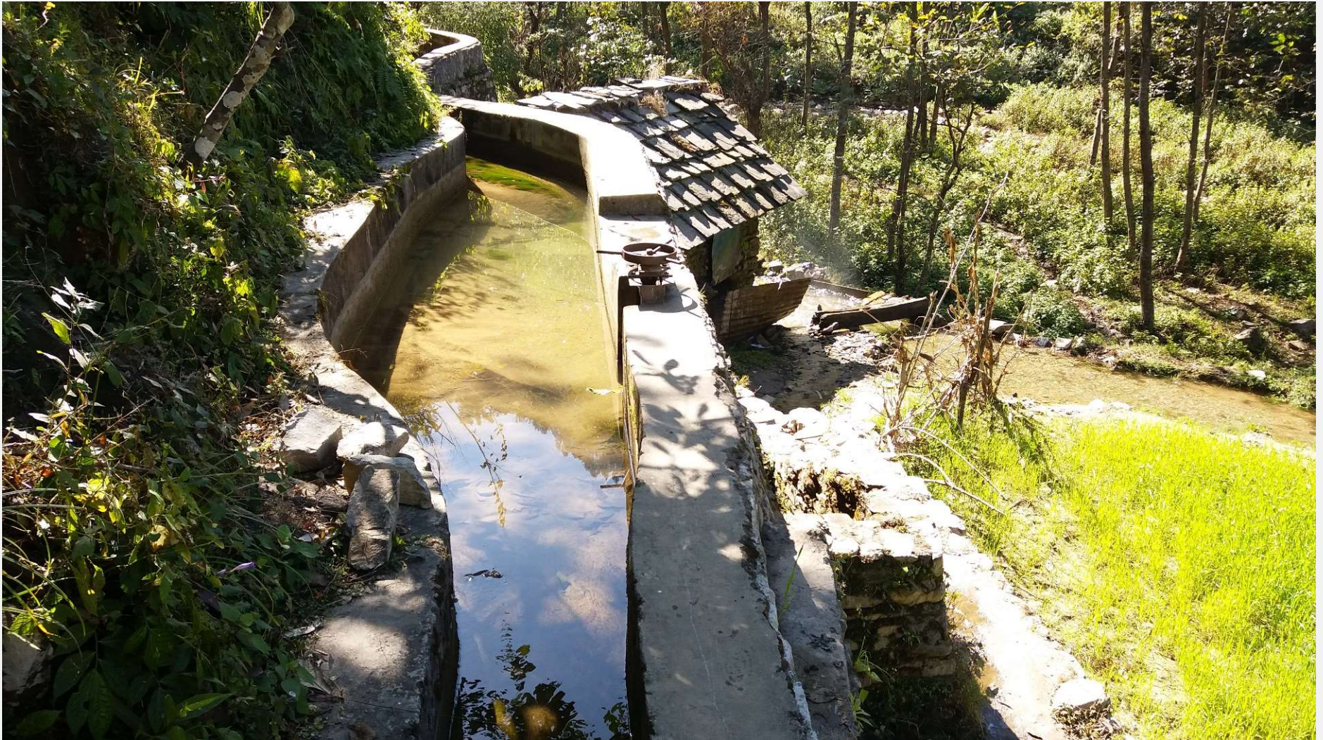
Gravel Trap/ Settling Basin
